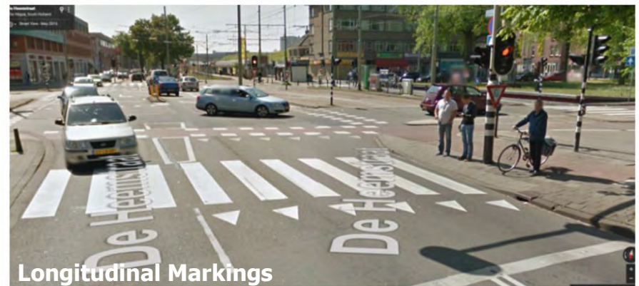
Colored Textured Pavement with Shark Teeth Markings
